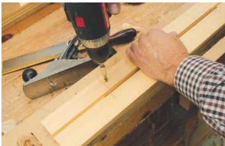
▲ Pic.10 ...then fasten the pocket piece back into its stile with a countersunk screw
